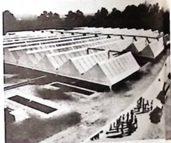
Solar collector panels mounted on roof of George Town's Elementary School in Atlanta, Georgia.
