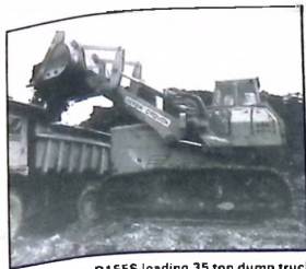
The Komatsu D155S loading 35 ton dump truck.
