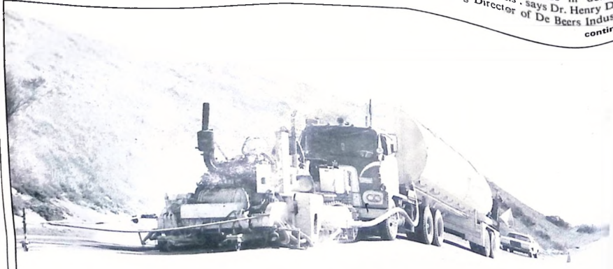
Grinding 'bumpy' concrete road surfaces flat and true, and generating anti-skid grooves in surfaces which have worn down smooth. This operation is carried out by special machines fitted with diamond blades. Mammoth 22,000 lb machine in the foreground is fitted with 265 diamond cutting blades. Behind the machine is a water tanker for cleaning the road surface.
