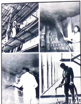
The "Turbosol" concrete spraying machines with built in mixer to mix and spray mortar or plaster onto walls.
