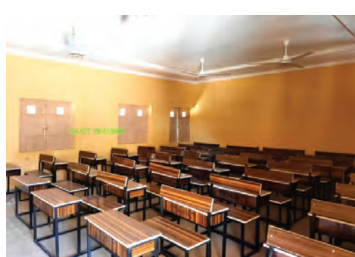
Newly completed and furnished classroom at GGC Damaturu
