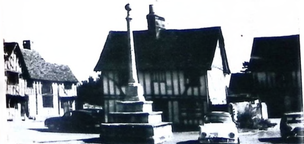
"Elizabeth's sturdy burghers tarred the oak framework of their half-timbered houses to such good effect that many of them are still lived in" Lavenham in Suffolk, UK. (photograph Noel Moffett)
