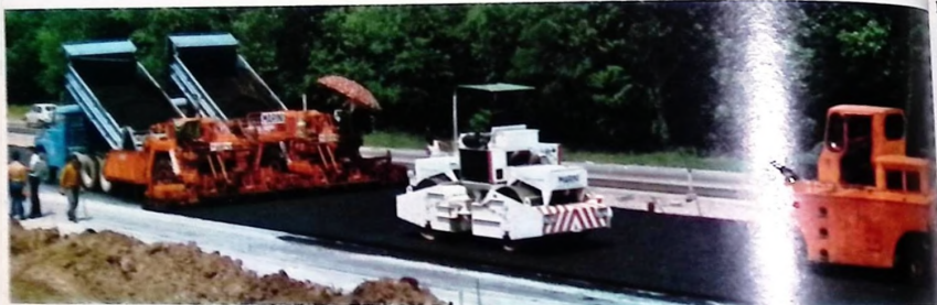
Finishers (tyred and tracked)
