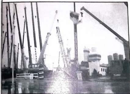
Central view of the Coles stack handling (centre) Coles Hydramobile 911 and (centre left) Coles Hydratruck 12/14T 4 x 4
