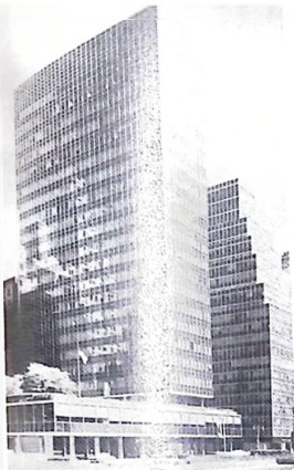
Lever House, New York. Fine example of modern glass curtain wall construction.
