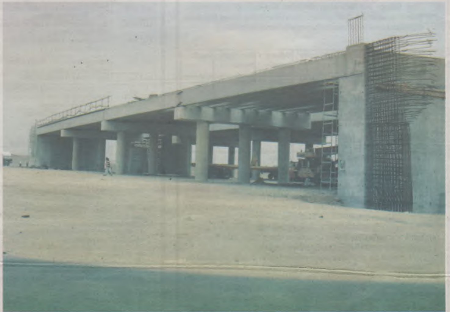
AN interchange under construction along the Abuja airport road
