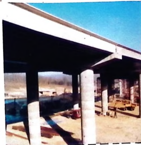
Prestressed concrete slab for tramway track construction system.
