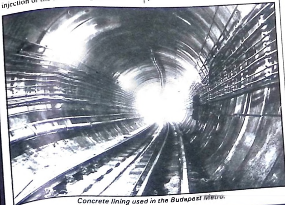
Concrete lining used in the Budapest Metro.
