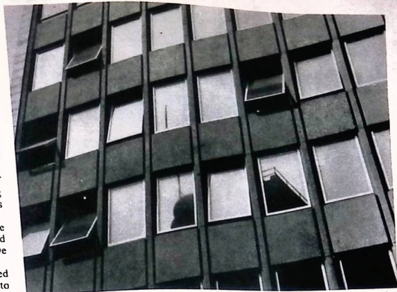
A good example of hardwood window frames which are widely used in colleges, schools and research laboratories
