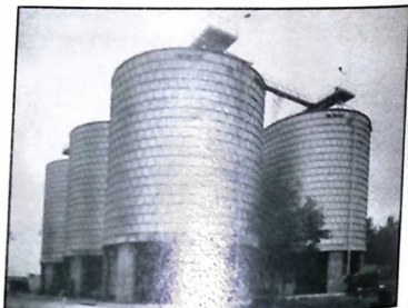
A group of silos for grain storage.
