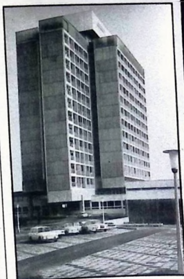
The frame of this modern hotel was built in precast concrete manufactured by a special process developed by UNIVAZ.
