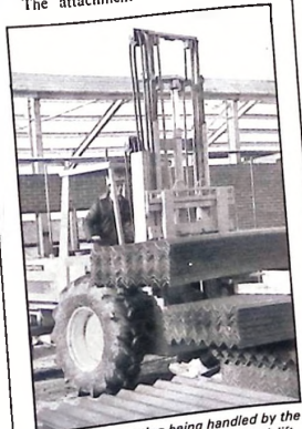
Corrugated sheeting being handled by the International Harvester 2525 fork lift.
