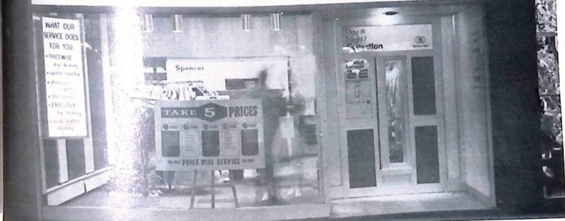
The front view of a very modern unit cleaning shop with a Spencer machine in the background. The automatic device on the right permits customers to collect garments at any time of the day or night by insertion of a pre-paid control card. The unit automatically identifies individual garments from storage rails.
