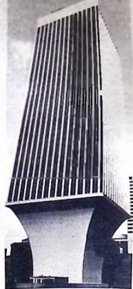
BALANCING ACT — The Rainier Bank Tower in Seattle, Washington, not only has the townspeople talking but also has them looking up nervously as they walk past. Measuring 40 meters wide, the tower is balanced on an 11-storey concrete base that narrows to just 21 meters wide at street level. This makes the entire building look as if it is about to tip over.
