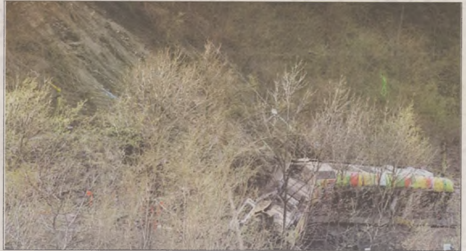
MUD and debris from the landslide can be seen on the hill above the tracks, where the wreckage of the train lies with the front carriage dangling out over the River Adige
