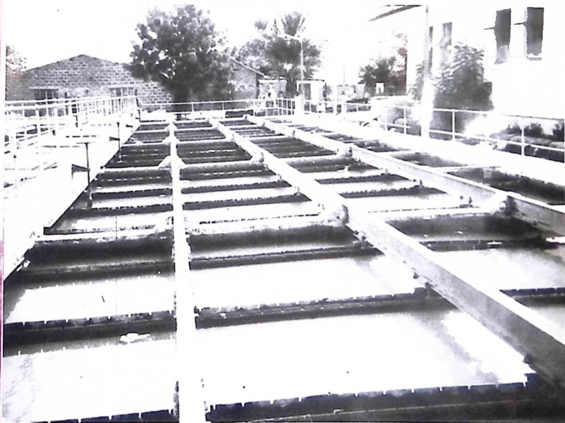
One of the Water treatment plants at Chalawa Dam. Sarkin Kano Alhaji Abdullahi Bayero constructed the Dam. The project started in 1927 and completed in 1930. The Dam is still functioning, and maintained by Kano State Water Board.
