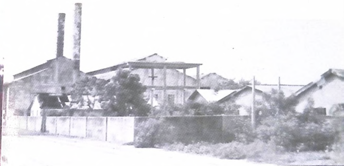
The remnants of Thermal Electricity Generating Plant constructed by Sarkin Kano Alhaji Abdullahi Bayero at Chalawa. It was completed and commissioned in 1929. This power station supplied the whole Kano and its industries with uninterrupted power supply.
