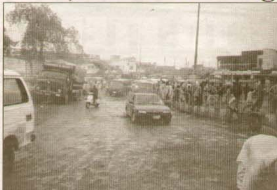
One of the worst affected roundabouts in Kano, Yankura roundabout, flooded due to lack of proper drainage.
