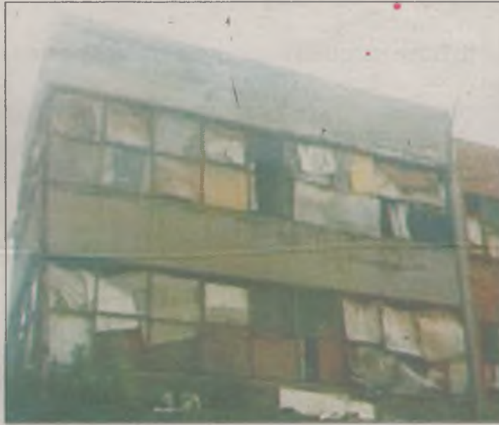
THE building is now completely derelict
