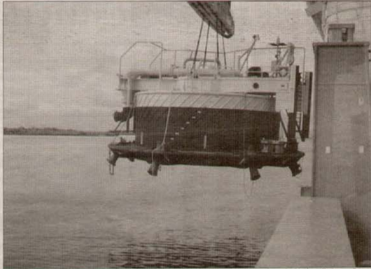
New loading facility, Calm Buoy, which is used to load crude oil to Ocean-going tankers, during installation at Bonny Terminal...recently.
