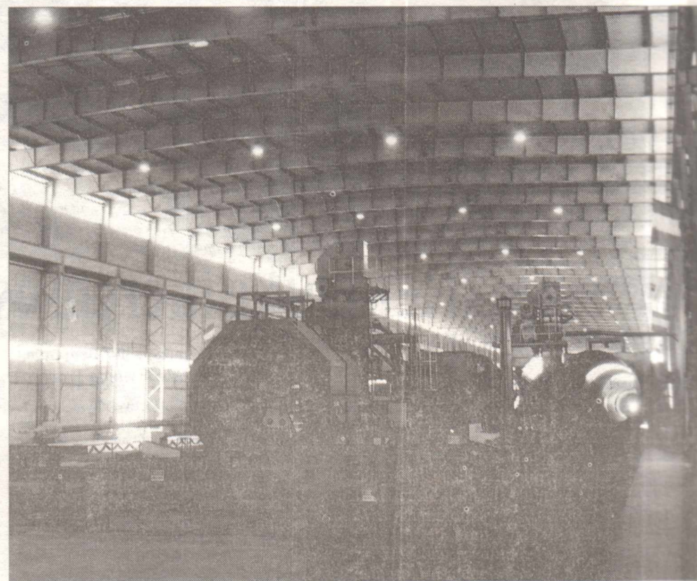
The newly commissioned SCC Steel Water Pipes factory commissioned by President Olusegun Obasanjo in Abuja last Friday
