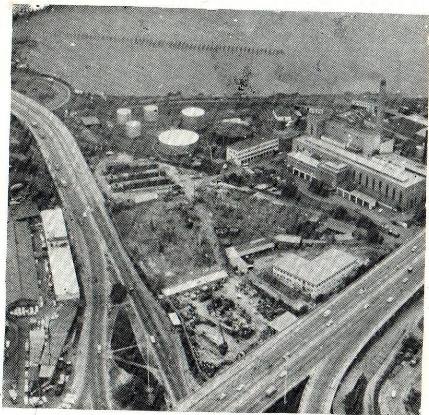
Part of the ring road linking different parts of Lagos
