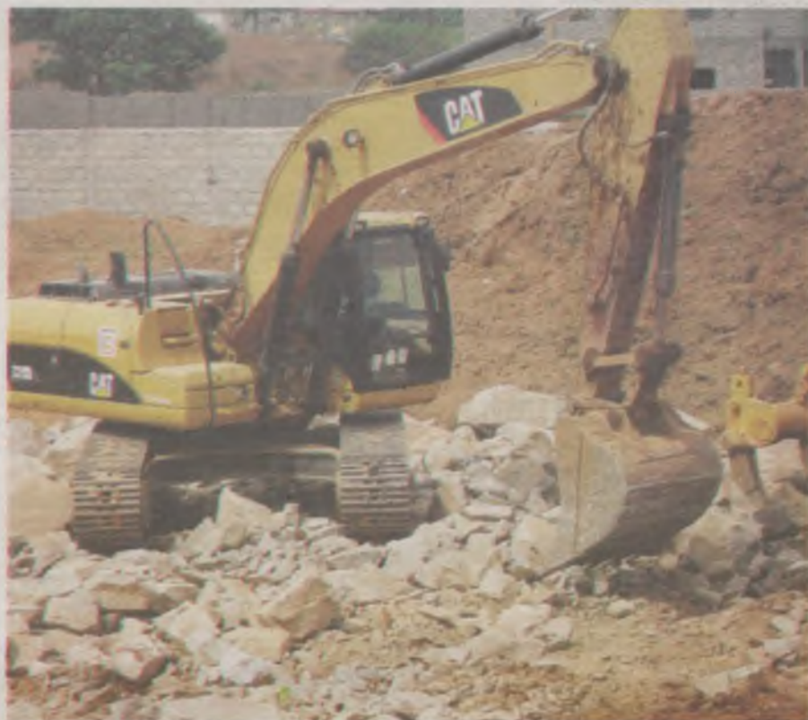
WORK in progress at the Kubwa expressway expansion project site
