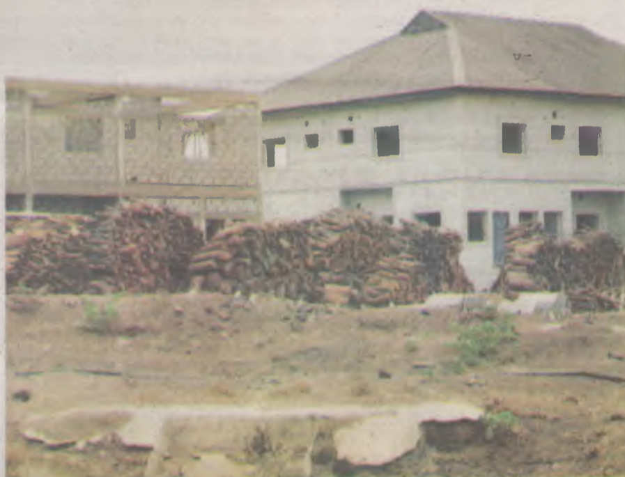
HOUSING development by the FHA in Gwarimpa Housing Estate, Abuja
