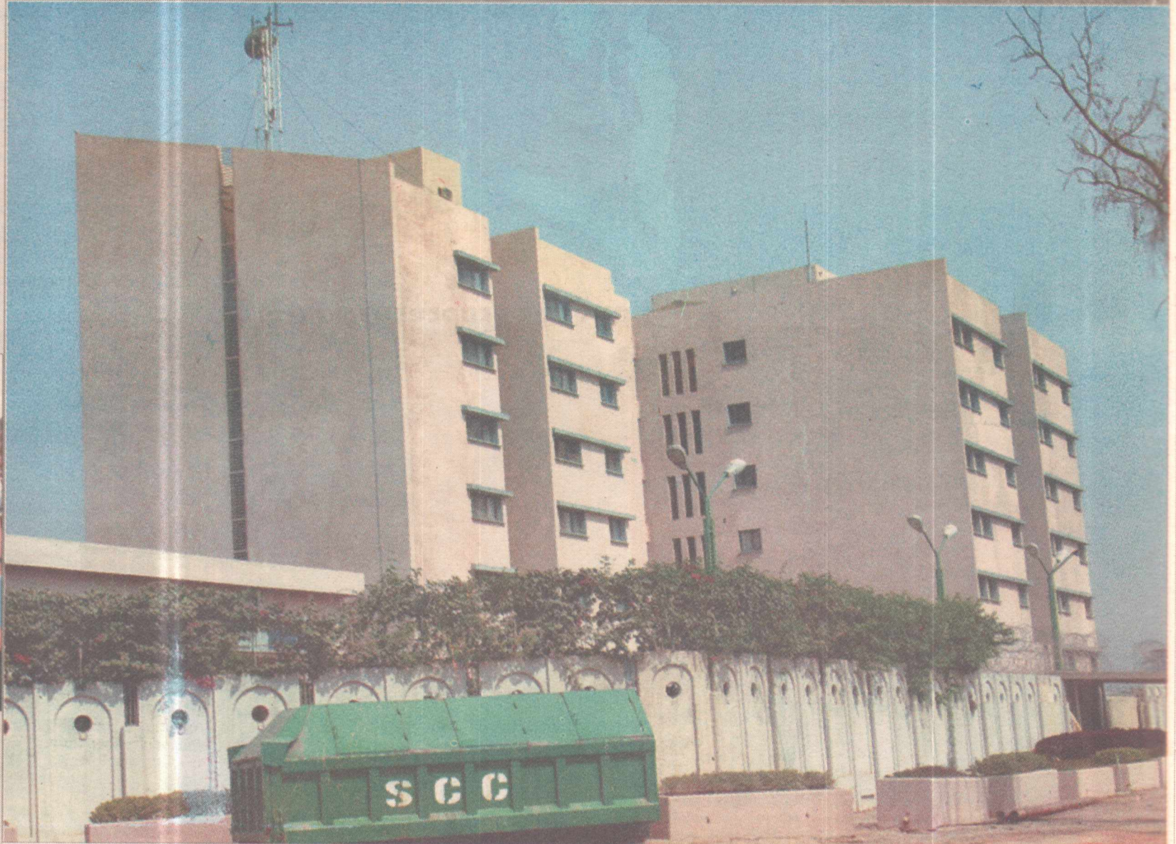
The SCC Headquarters complex: The SCC (Nig) Ltd headquarters complex is a tastefully designed structure situated within the Utako district of Abuja FCT.
