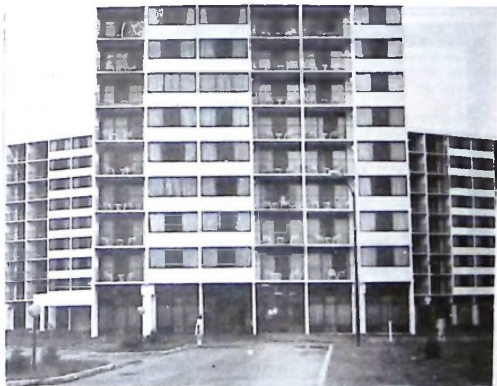
One of Government's housing projects in the capital.
