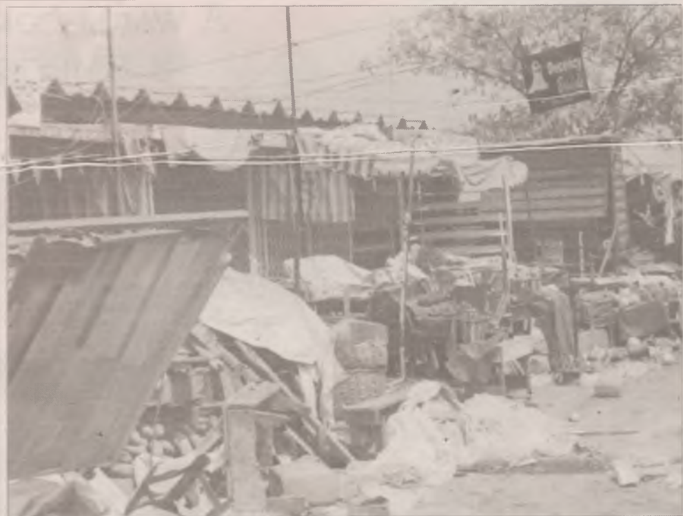
Some of the demolished shops at the Wuse Old market...last week.
