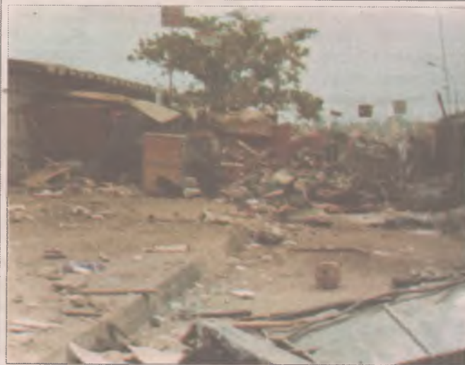
Another section of old Wuse Market after the demolition...last week.
