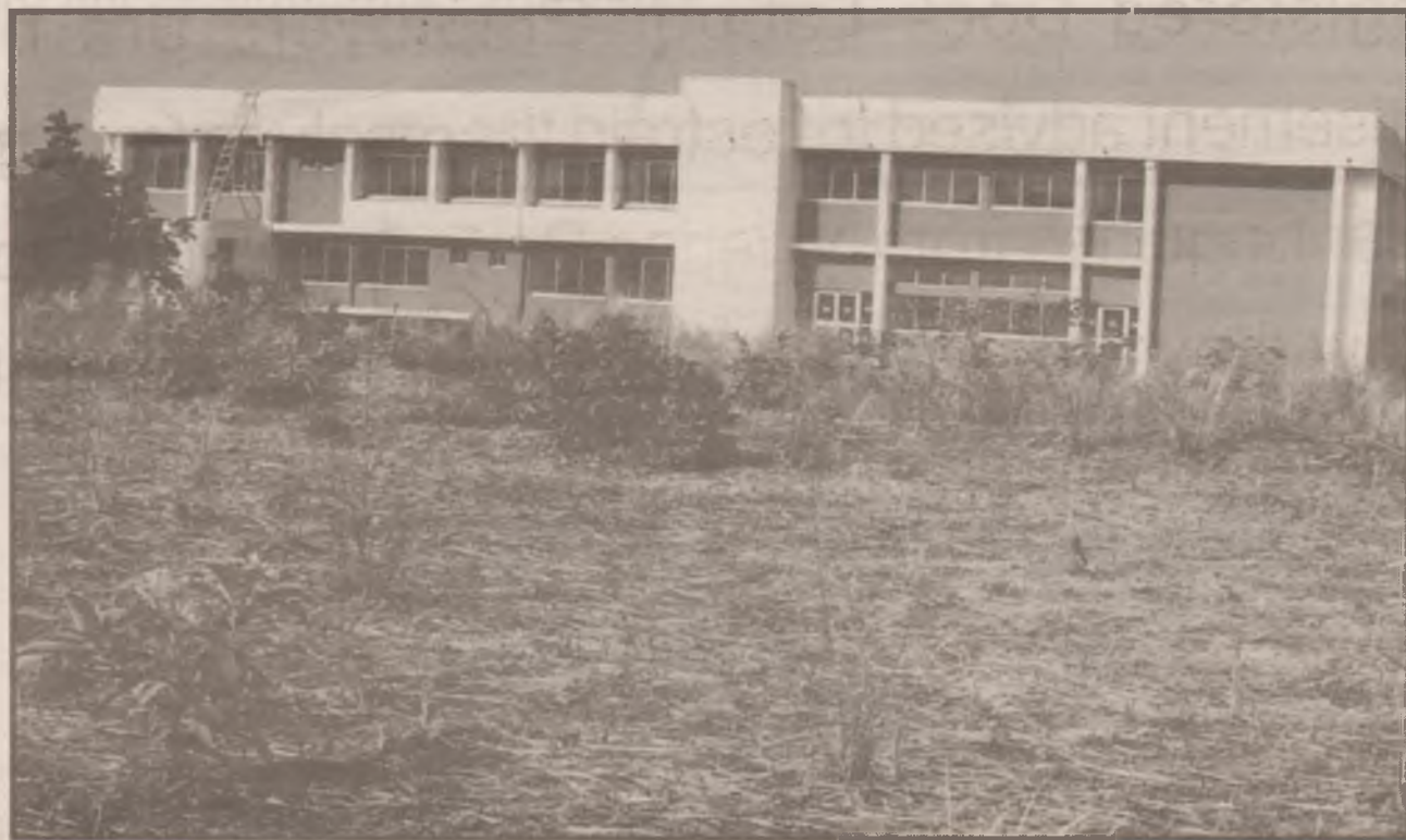
A completed court complex in Gwagwalada that needs to be connected with light, water and an access road.
