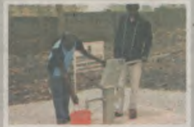
Borehole at Christian Association of Nigeria [CAN] Headquarter, Kaduna State Chapter
