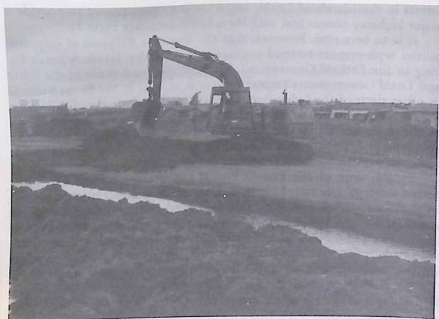
Plate 1: Construction Work on Ibeju-Lekki Highway.
