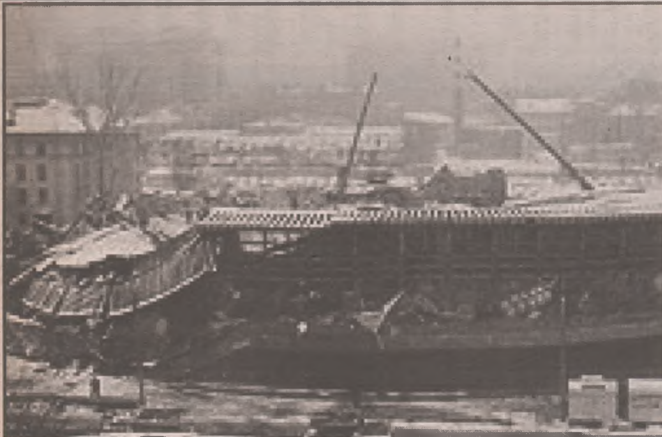
Market traders were setting up when the roof collapsed.
