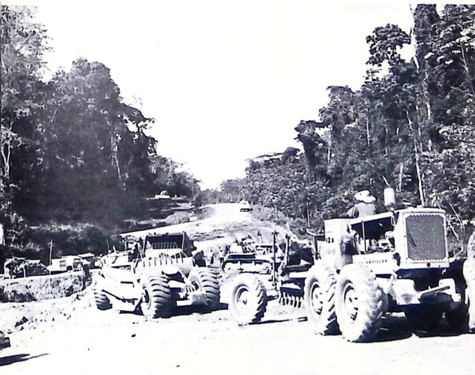
Road construction in progress.
