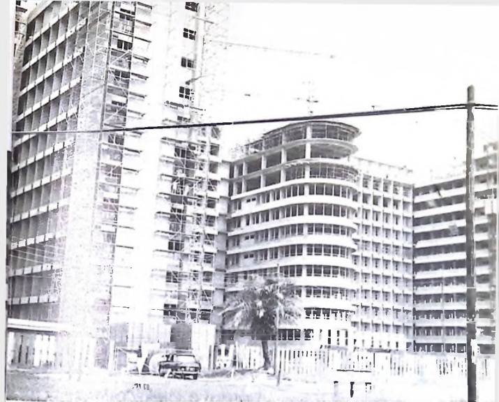
The new Federal Secretariat, Lagos, under construction.
