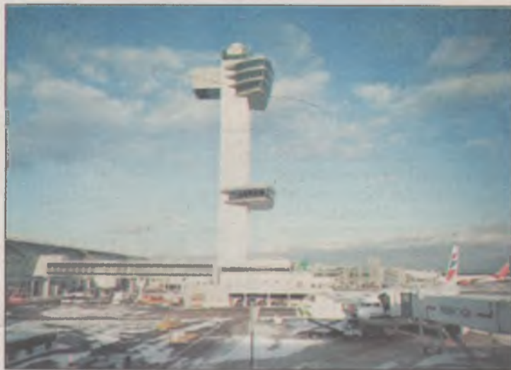
THE air traffic control tower at JFK airport in New York where a child was heard directing planes
