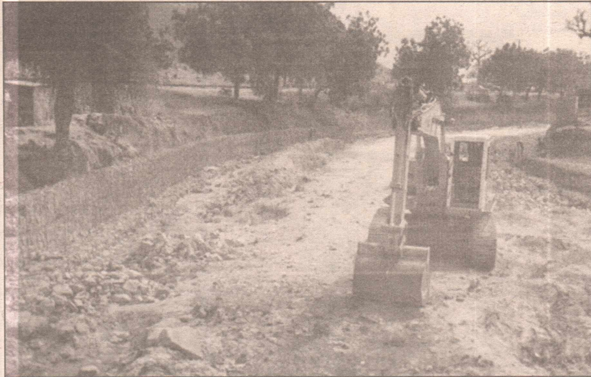
Erosion control to make rural infrastructure more long lasting
