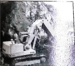
Demag's H71 excavator ideal for queue work
