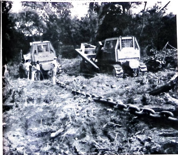
Clearing land with heavy equipment in northern Ivory Coast
