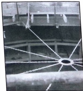
Inside view of the slipform
