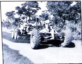
A caterpillar grader at work improving the roads
