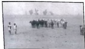
A view of the dried-up river bed which produced raw materials for the batching plant on-site.
