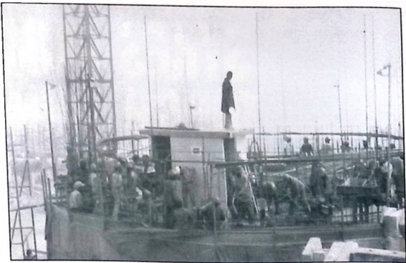
Working on the slipform
