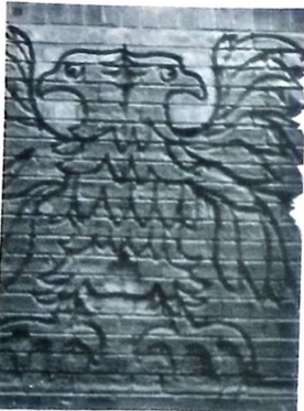
Contrasting flush and raked-out mortar joints on a church in Birmingham, UK designed by John Madin Design Group
