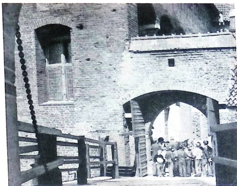
This size of brick (225 by 112½ by 75mm) has been used throughout the history of architecture. A mediaeval town in Poland.
