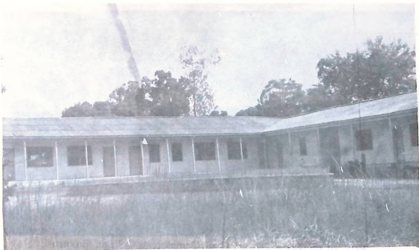
Part of the Classroom Buildings of Simmats Jos.
