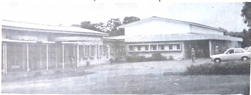
The out Patient Department of the Murtala Muhammed Hospital, the largest Hospital in Jos.
