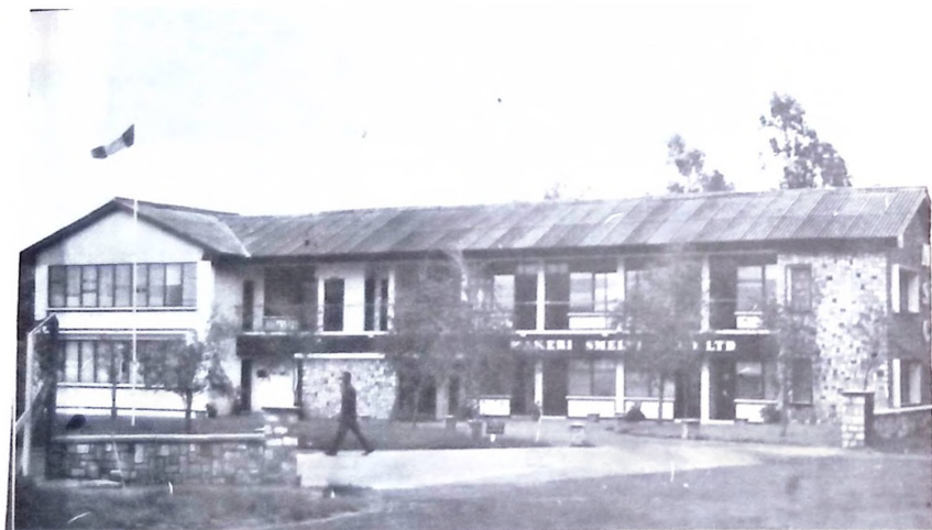
The Administrative Block of Makeri Smelting Company Ltd.
