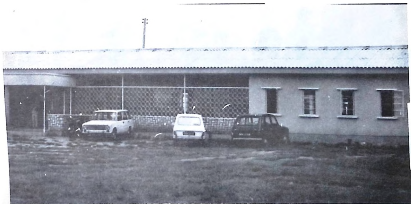
The Administrative Block of the Government Staff Training Centre, Jos.
