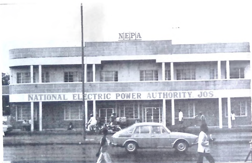
Offices of the National Electric power Authority, Jos.
