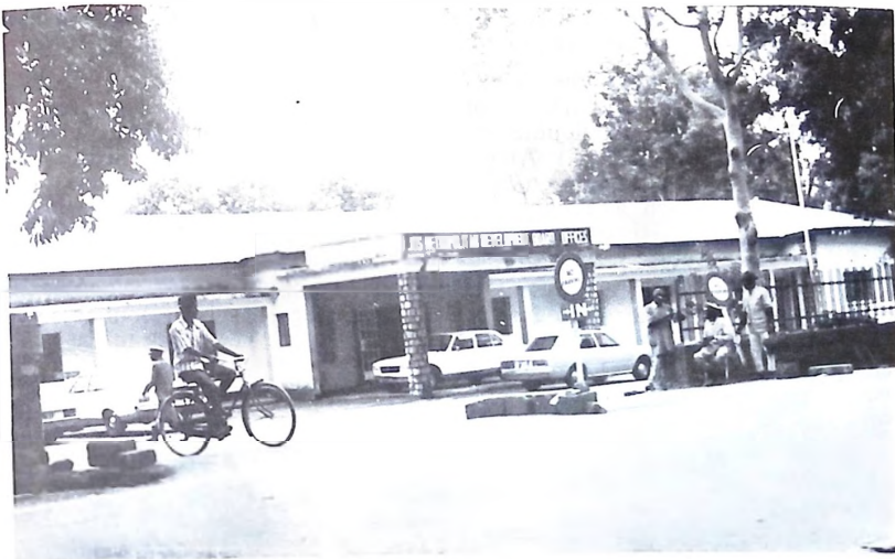
Offices of the Jos Metropolitan Development Board.
