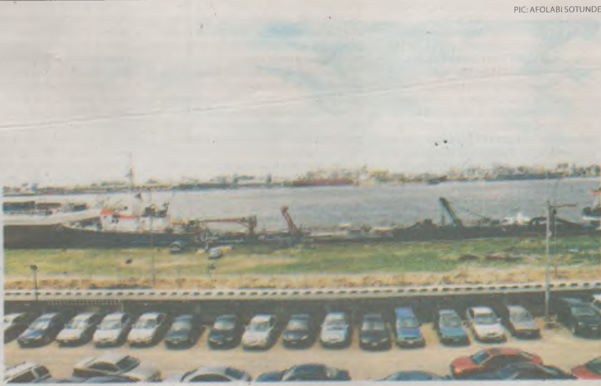
APAPA wharf, Lagos, viewed from the Marina.
