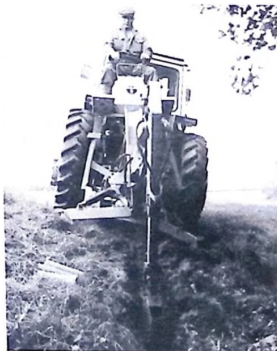
McConnell Power Arm 8, demonstrating self-leveling capacity - a useful attribute in trenching work. The PA8's tilting king post and hydraulic stabilisers ensure vertical trench sides despite sloping terrain.
