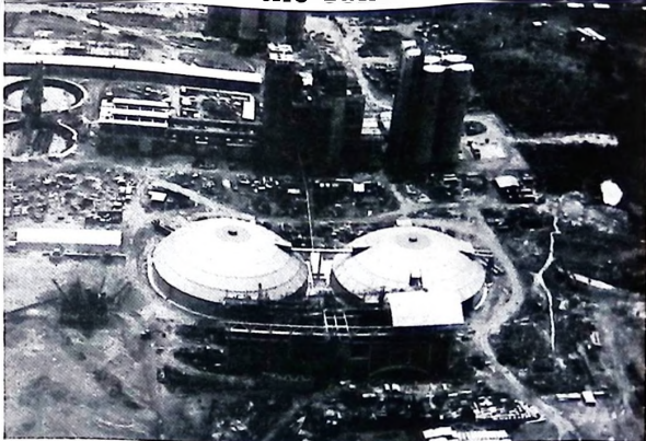
Overview of Benue Cement Works during final stages of construction.
