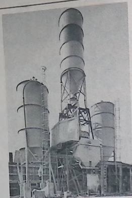
Brun concrete batching plant
