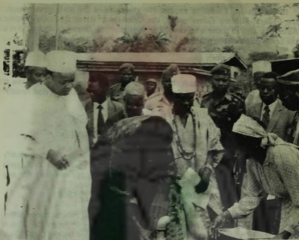
Commissioning of Federal Government borehole project at Imesi Ile by Col. Oresanya
