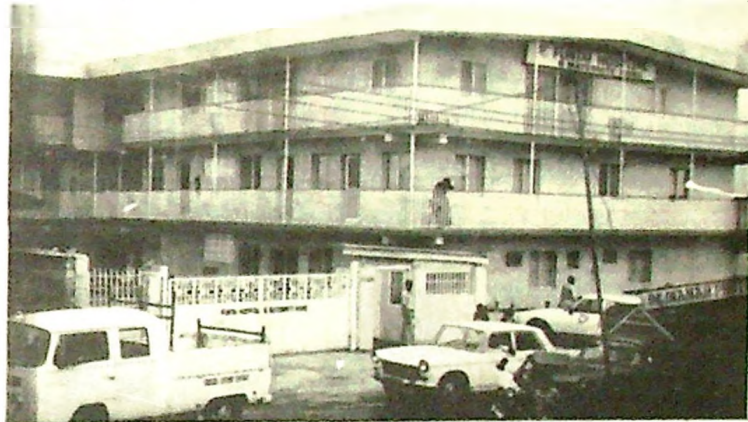
FUNTAI HOSPITAL COMPLEX
