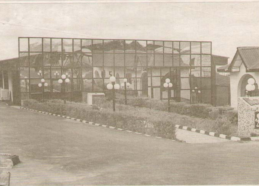
The 1000 seater valley view auditorium built in eight weeks by the Ogun State government.
