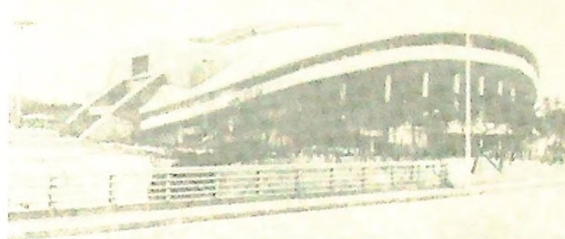
• Olympic indoor swimming pool in which synchronized swimming and water polo events will take place. The last main games site to be completed this month.
