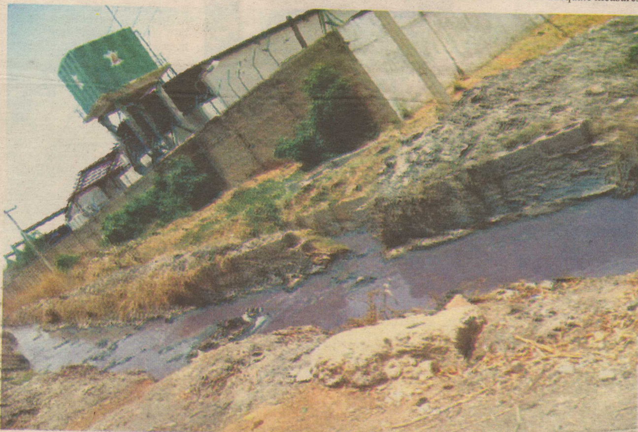
This waste which originates from one of the industrial estates empties into the Kano River
