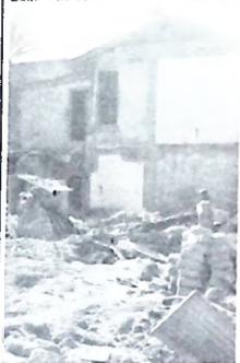
• Devastation: Houses destroyed by the flood
