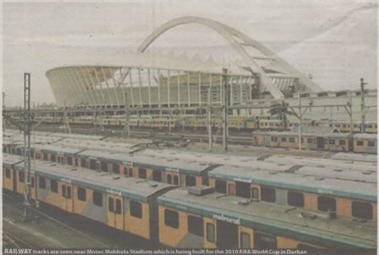
RAILWAY tracks are seen near Moses Mabhida Stadium which is being built for the 2010 FIFA World Cup in Durban
