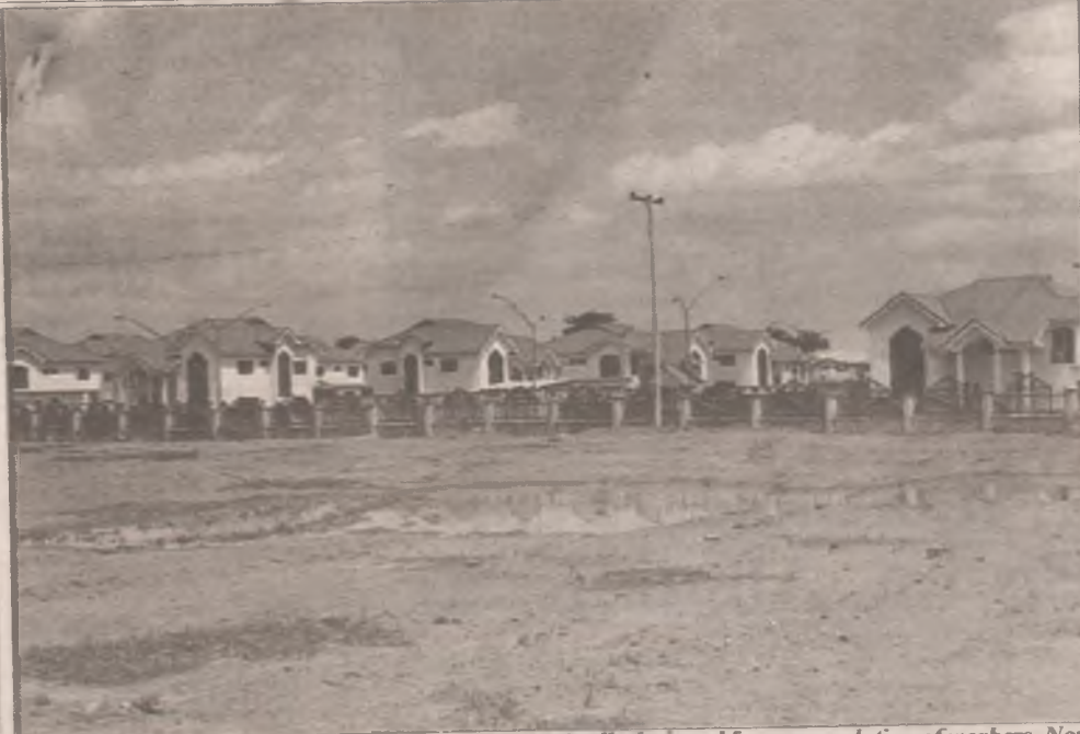
Houses at Gwarimpa estate in Abuja. They were originally designed for accommodation of workers. Now government has decided to sell them to those who can afford to pay. When will the average Nigerian worker ever get decent and convenient accommodation? Pix: Felix Onigbinde
