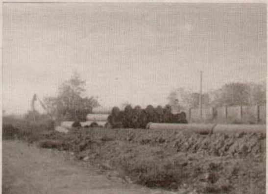
The huge pipes imported by Former Kano Governor, Rabiu Musa Kwankwaso wasting away by the road side in Kano.
