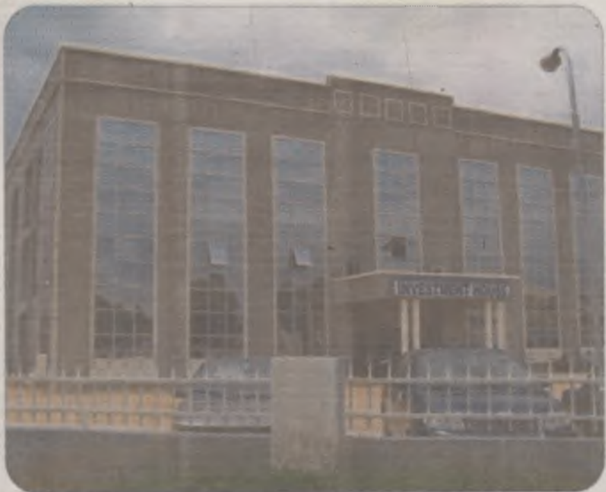
Newly constructed Headquarters complex of the Nasarawa Investment and Property Development Company (NIPDC) along Jos Road , Lafia.
