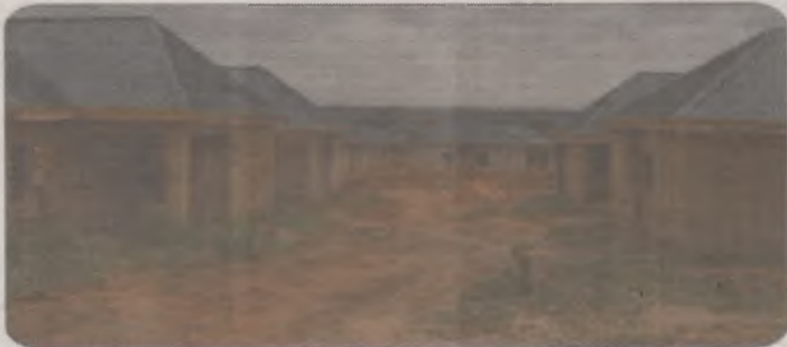
Second phase of the 500 Housing Units for civil servants in Lafia
