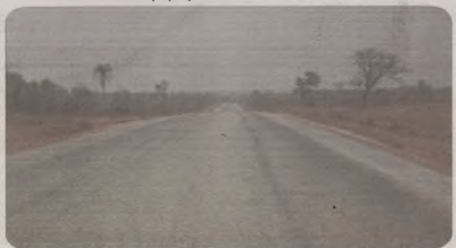
Nasarawa Eggon-Mada Station Road is one of the 12 major road constructions embarked upon by Gov Doma aimed at opening up the state for effective communication and to stimulate business activities.
