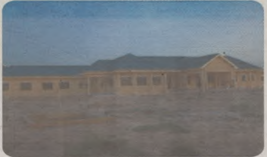
One of the newly constructed complex, providing-office accommodation for some of the ministries in Lafia.
