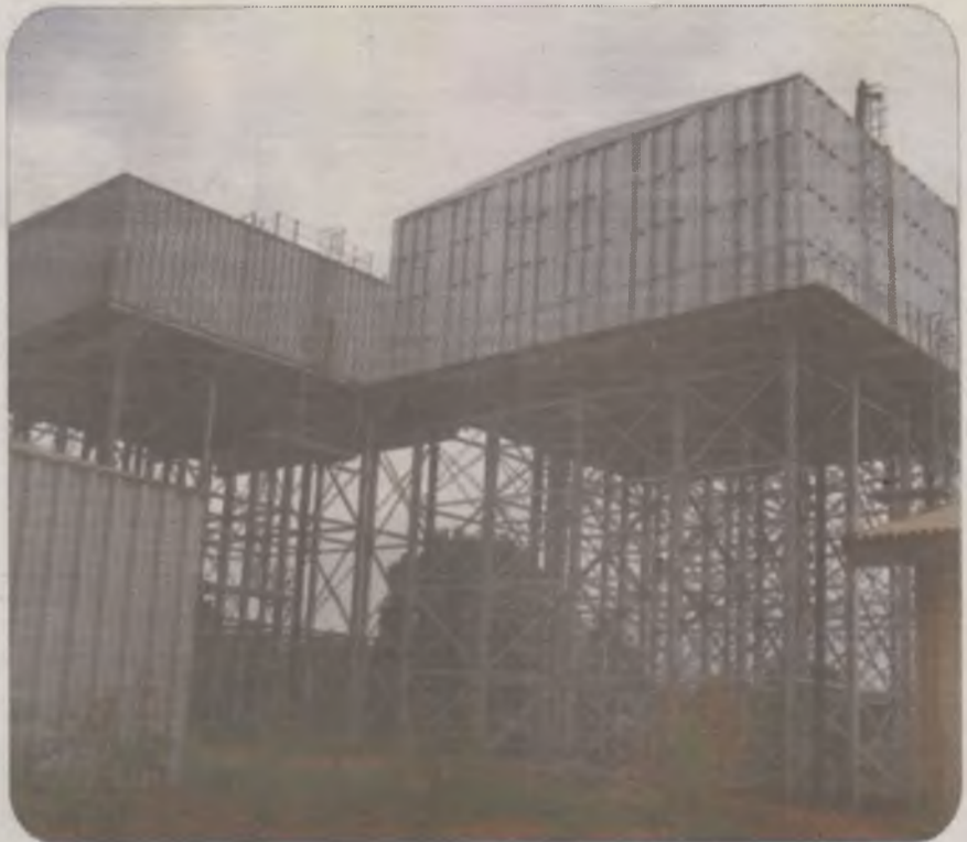
Expansion and upgrade of water scheme in Lafia completed and waiting commissioning.
