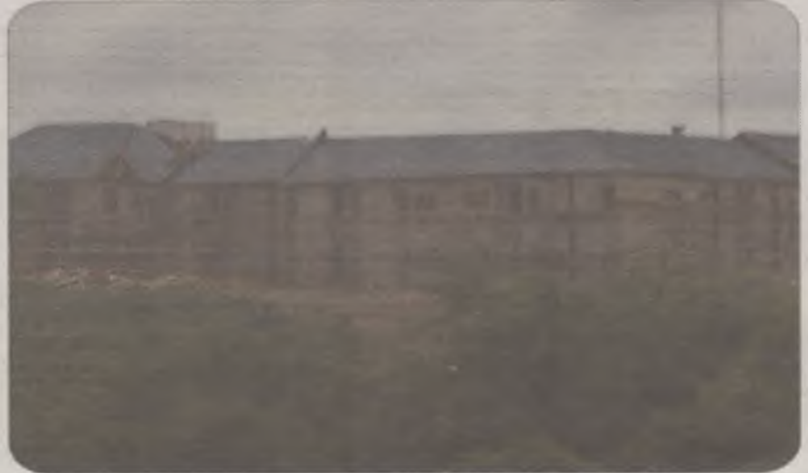
Hostel accommodation for School of Nursing and Midwifery, Lafia under construction.
