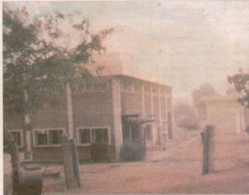
The power house of one of the dams, the difficulty in getting drinking water from other sources is usually at its peak there. The water is served that country under a bilateral agreement with Nigeria.
