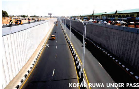
Late Alhaji Tijjani Hashim Underpass along Katsina Road
